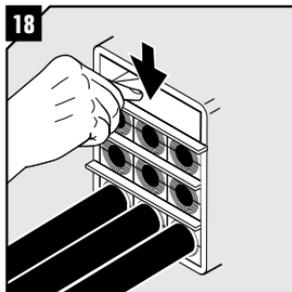
Separate the two stayplates and insert the final row of modules between the stayplates. Drop the upper stayplate on top of the modules.
