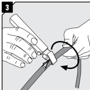
Cut the outer sheath with a tool of your choice. Make sure not to damage the cable screen.
